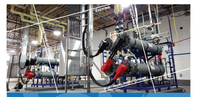
De Nora ClorTec<sup>®</sup> and MIOX<sup>®</sup> On-site Chemical Generators
